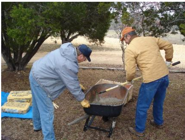
Jim Hillin and John Pratt mixing concrete
