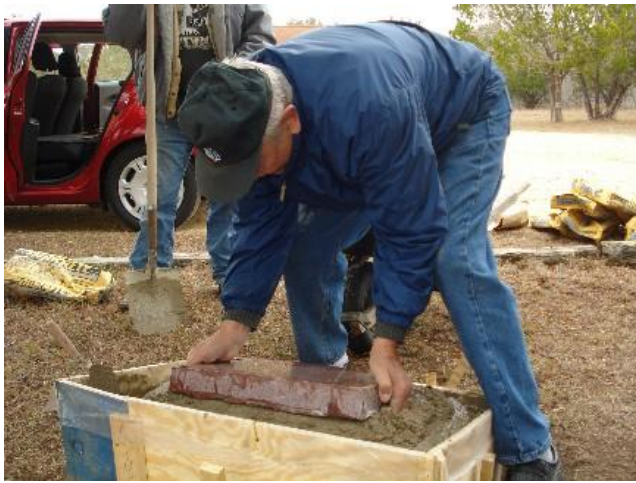
Huber Dirr working the concrete into the mold
