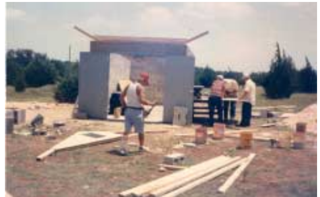
Rick Compton and many club members helping with the construction
