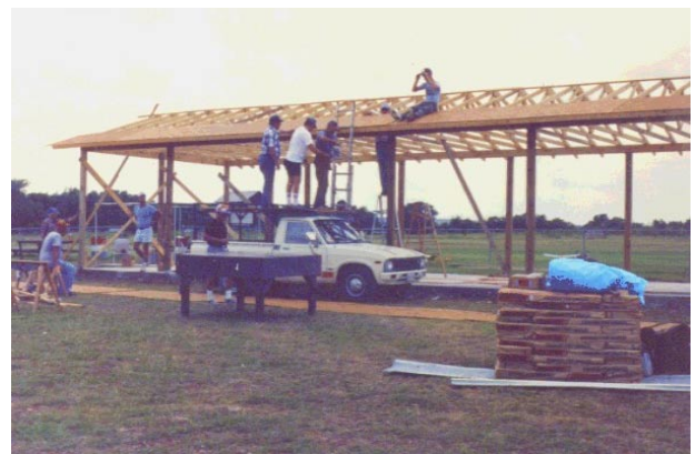
SHINGLES HAVE BEEN DELIVERED
