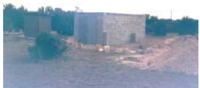
The walls are up and ready for the roof
