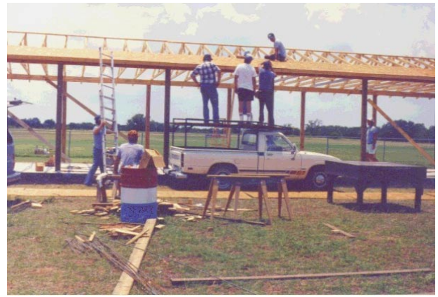
RAFFTERS UP AND DECKING BEING LAYED
