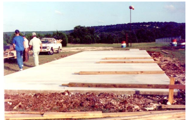
CONCRETE IN AND POST BEING LAYED OUT
