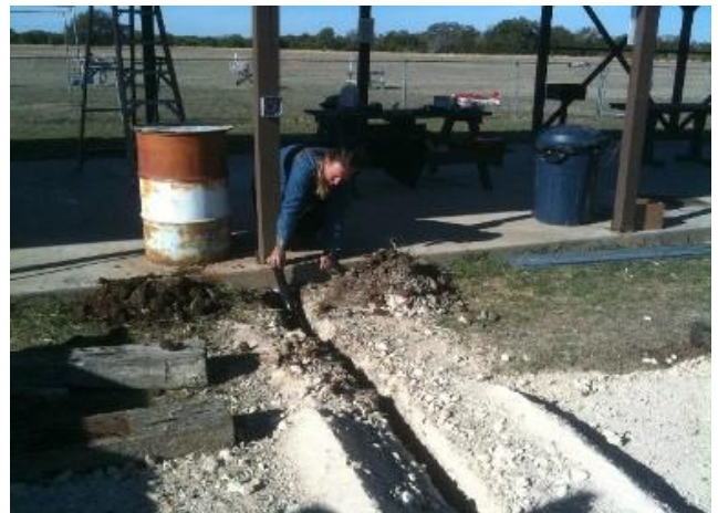
Fred Gortler laying pipe
